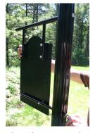
Insert hanger arm rods into sign post. Thread 1/2" stainless machine screws using an Allen wrench through post wall.
